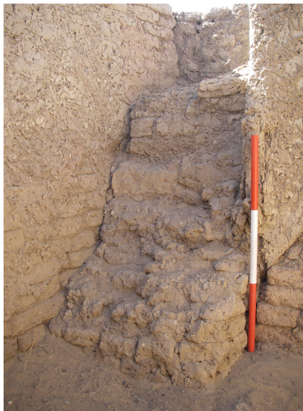
Plate 3: view of staircase in room A32 (to W).
