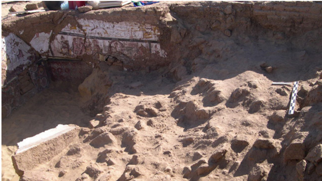
The collapse of the dome in the original Villa.
