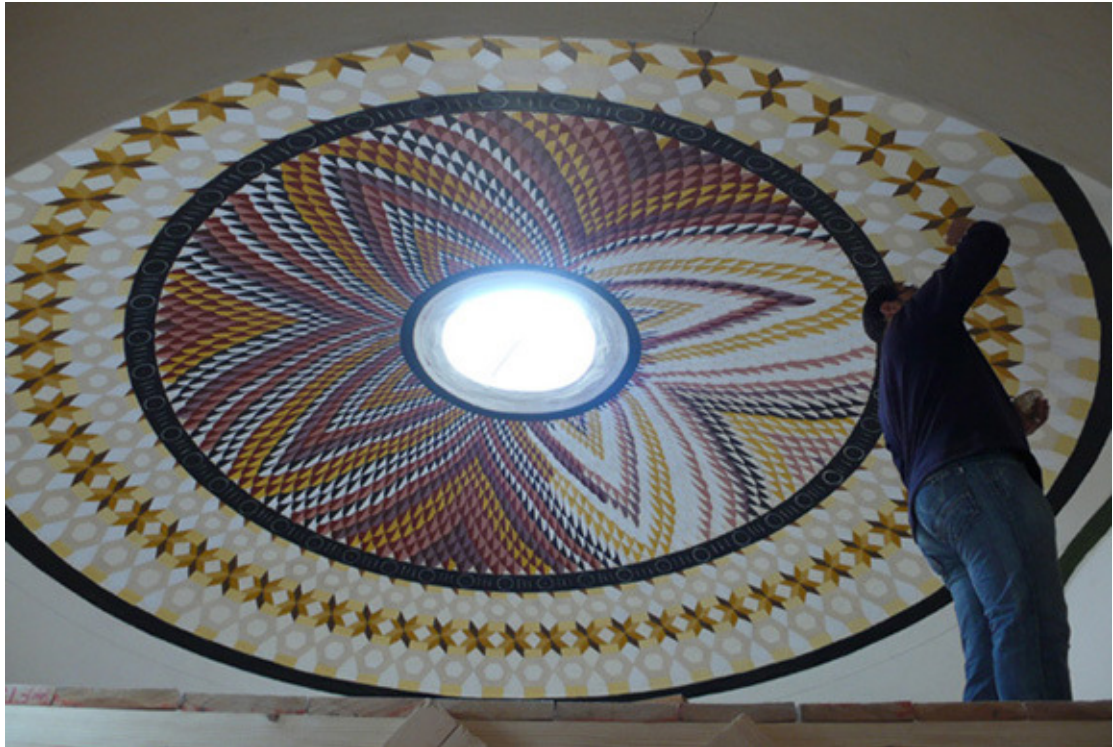
Tamer painting the first layer of colours for the 'coffering'.
