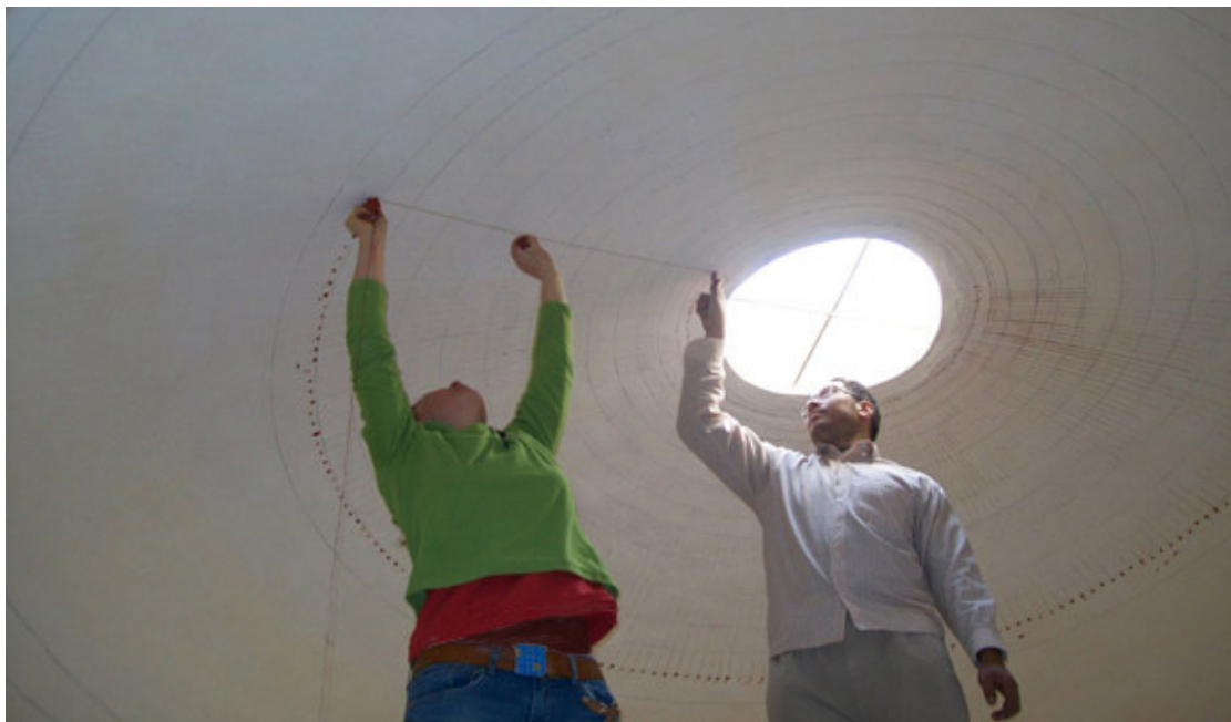
Setting up the grid with a chalk line - a piece of string, dripped in red colour. It has to be 'fixed' on two points, then let it snap. The result will be a red line.
