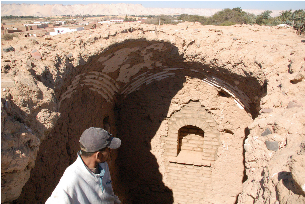
DOME AT HIGH LEVEL WITH RECONSTRUCTED NICHE ON NORTH WALL
