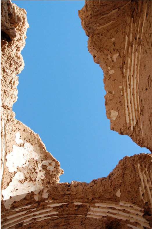
DOME BEFORE CONSOLIDATION
