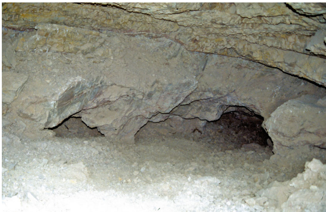
Fig. 5.174 New Kingdom mine at Dungash enlarged with a dome-like ceiling structure in the Ptolemaic Period, which significantly increased its stability
