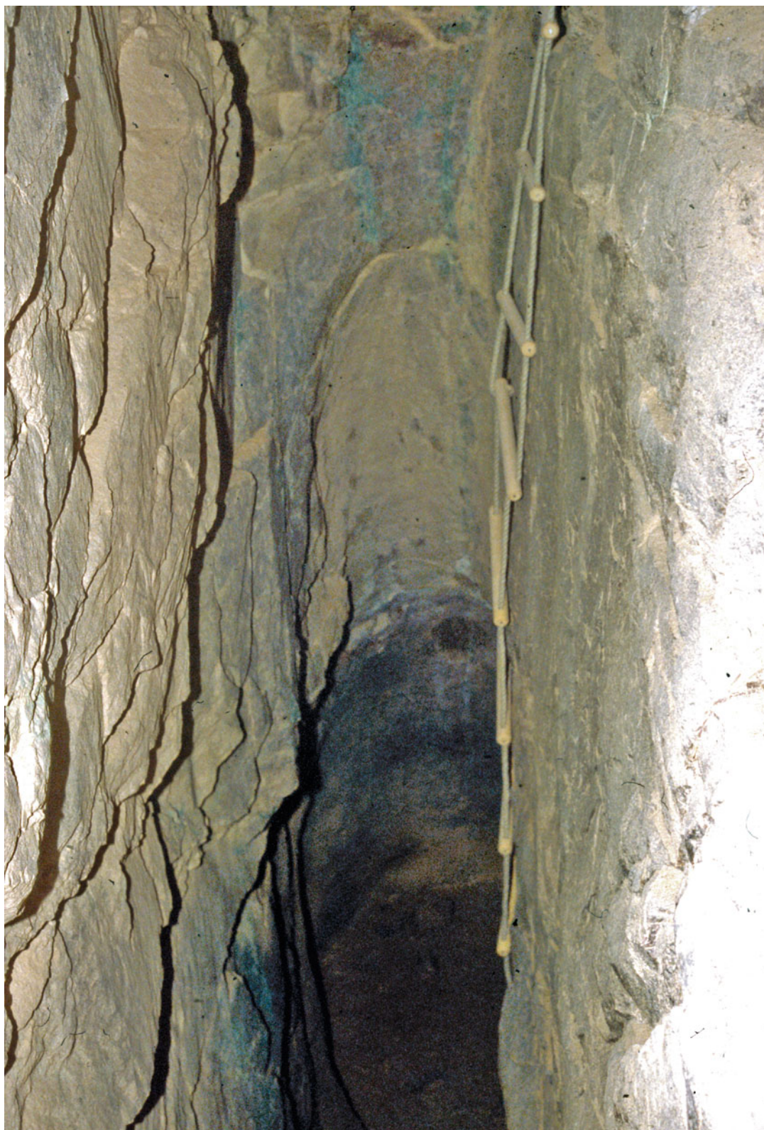
Fig. 5.127 Old Kingdom mine in upper Wadi Bokari with smoothed walls from the crushing effect through the use of heavy and blunt hammers
