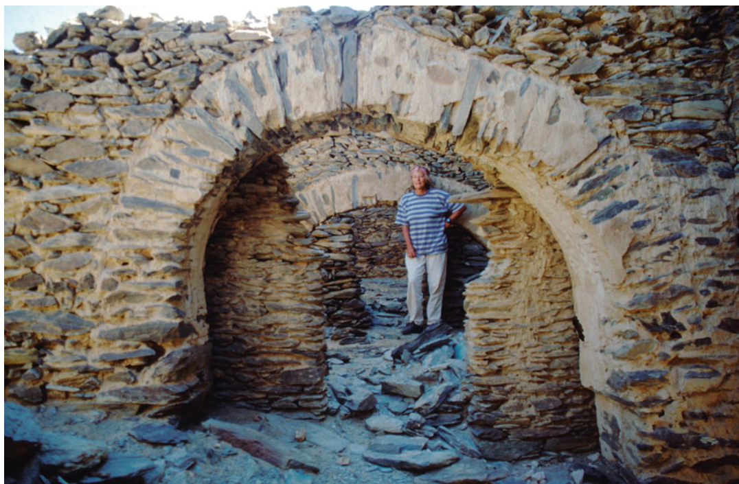
Fig. 6.98 Vaulted passageways inside the northern fort at Derahib. Note the clay mortar and remains from wall plaster
